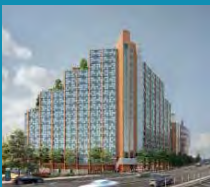
161 Talgarth Road - Under Construction
