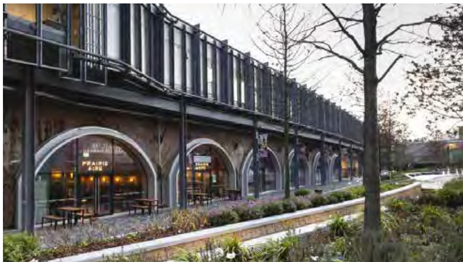
Renovated Railway Arches - White city
